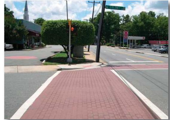
***Stamped and painted asphalt is one type of enhanced pavement used to highlight a pedestrian area.***
