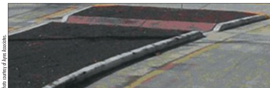
Figure 3. Barrier curb on the splitter island.
