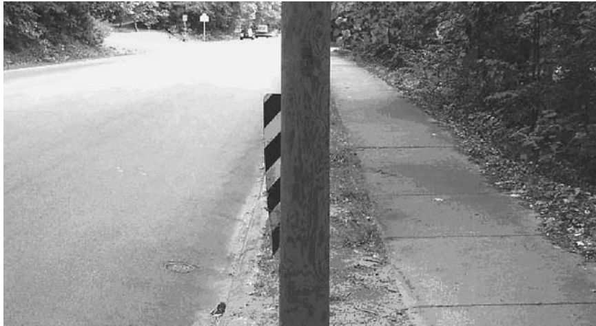
EXHIBIT V-13 New Pole Placed in Front of Object Marker An object marker failed to prevent the crash that took out the original pole it delineated. The new pole was placed in front of the object marker. (Photo: Brian Murphy)
