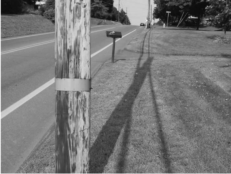
EXHIBIT V-12 Reflective Taping Used by Pennsylvania DOT
