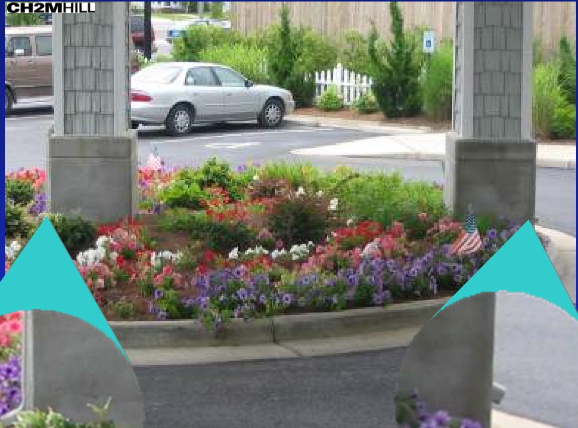
Roof Leader Disconnection (Chincoteage, VA)
