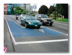
Example of a bike box in Vancouver, B.C. Note the short bike lane, which allows cyclists to safely advance to the box.
