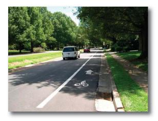
An example of a "road diet". This street was a four-lane street with a wide median. It was converted to a two-lane street, with bike lanes (and with the wide median remaining).
