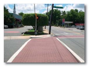
Stamped and painted asphalt is one type of enhanced pavement used to highlight a pedestrian area.
