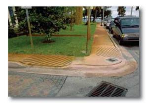
Two radically different curb radii. The radius at the top is very small (or "tight"), which helps to slow turning vehicles. The radius below is very large (or "wide"), allowing vehicles to turn more easily and quickly. Note the location of the crosswalk relative to the curve. The radius above is more conducive to pedestrian travel. Note also the different traffic characteristics - the intersection below must handle a much larger volume of traffic.
