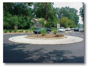
A roundabout in a residential neighborhood, where five street segments converge. Note the "apron" that allows larger vehicles to negotiate the roundabout.
