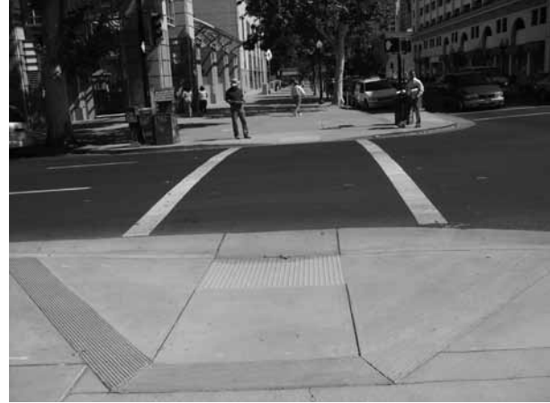
Figure 10.4 Intersections must be accessible to pedestrians with disabilities. This curb extension is equipped with curb ramps and high-contrast detectable warnings. Source: Kimley-Horn and Associates, Inc.
