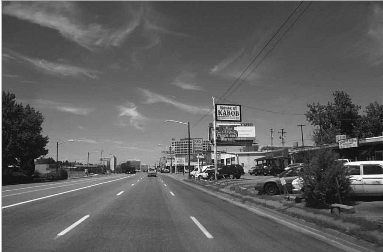
Figure 6.15 View of existing street. Source: Kimley-Horn and Associates, Inc.
