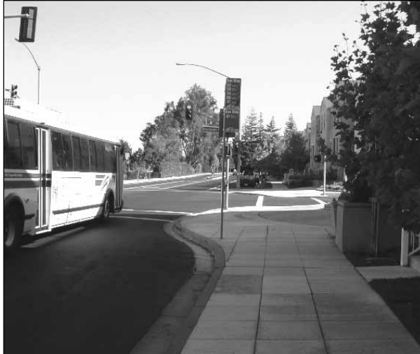
Figure 9.25 A typical bus turnout on an arterial Avenue. Source: Kimley-Horn and Associates, Inc.
