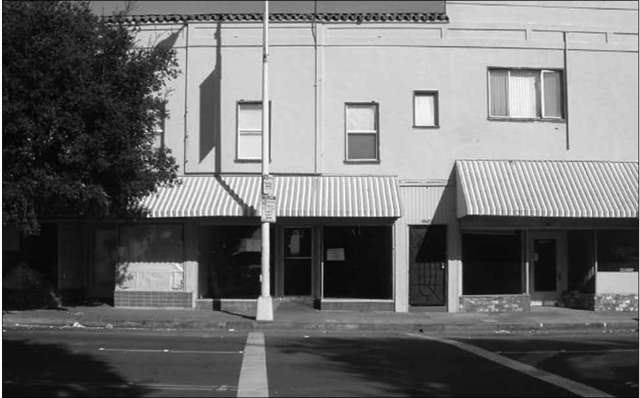
Figure 6.10 View of existing street. Source: Kimley-Horn and Associates, Inc.
