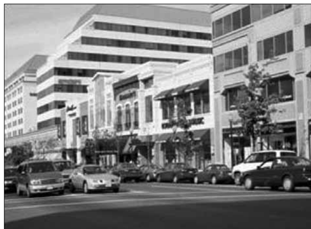
Figure 6.27 View of existing street. Source: Kimley-Horn and Associates, Inc.
