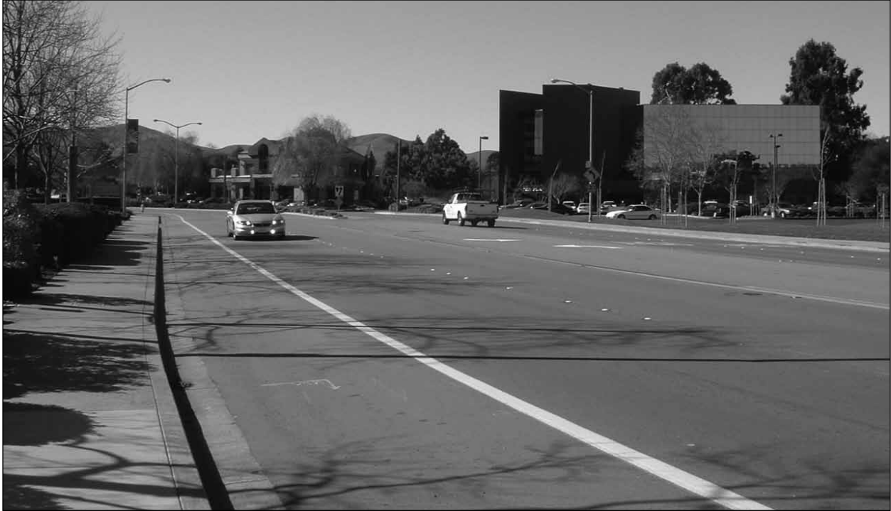
Figure 6.20 View of existing street. Source: Kimley-Horn and Associates, Inc.
