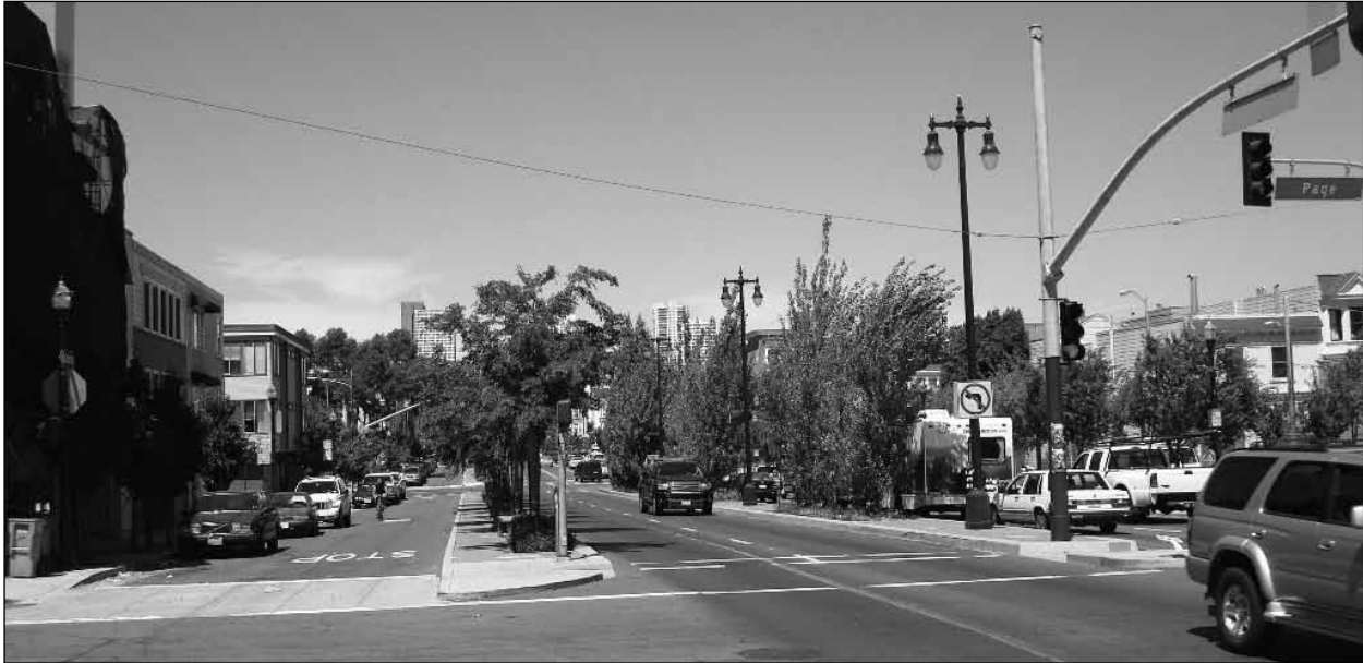
Figure 6.8 This multiway boulevard provides stop control for the low-volume, low-speed access lanes. The central roadway is controlled by a traffic signal. Source: Kimley-Horn and Associates, Inc.
