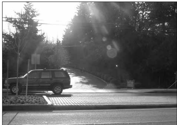
Figure 9.2 A mountable median allows emergency vehicles to access side streets. Source: Kimley-Horn and Associates, Inc.
