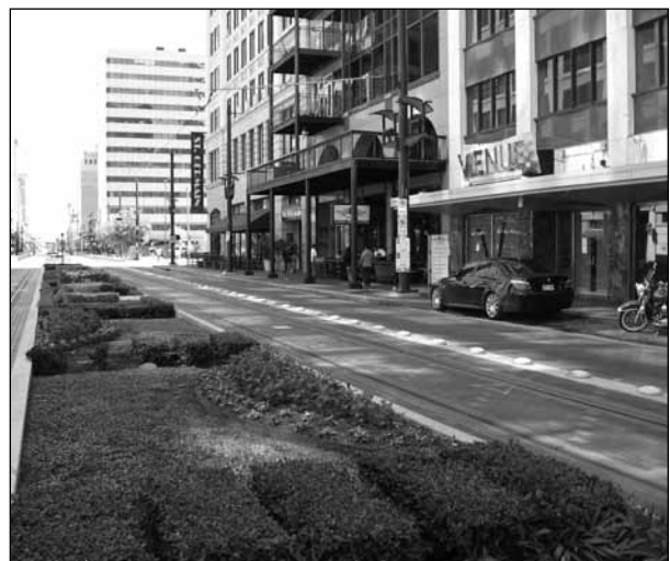
Figure 9.23 This thoroughfare in Houston, Texas has light rail transit running in dedicated inside travel lanes. Source: Texas Transportation Institute.
