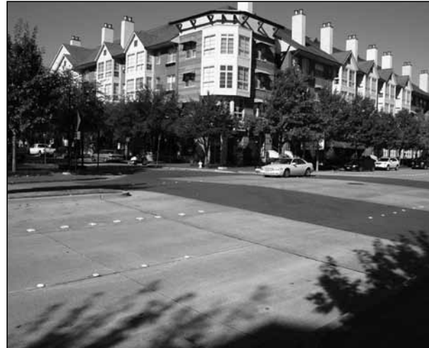
Figure 10.15 Crosswalks with colored bricks contrast with concrete pavement. However, over time, colored bricks stain and lose contrast. Painted stripes marking brick or colored concrete crosswalks would increase their visibility. Otherwise use standard crosswalk markings for long-term visibility. Source: Kimley-Horn and Associates, Inc.
